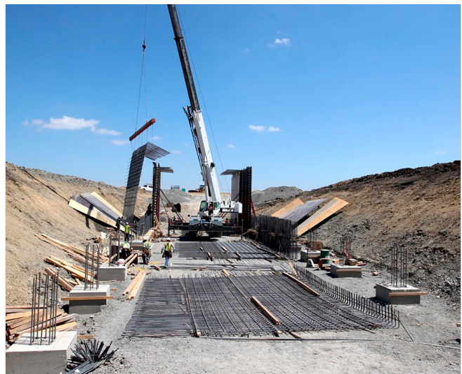
Construction of the Formula 1 racetrack. PHOTO: Courtesy of Circuit of the Americas
