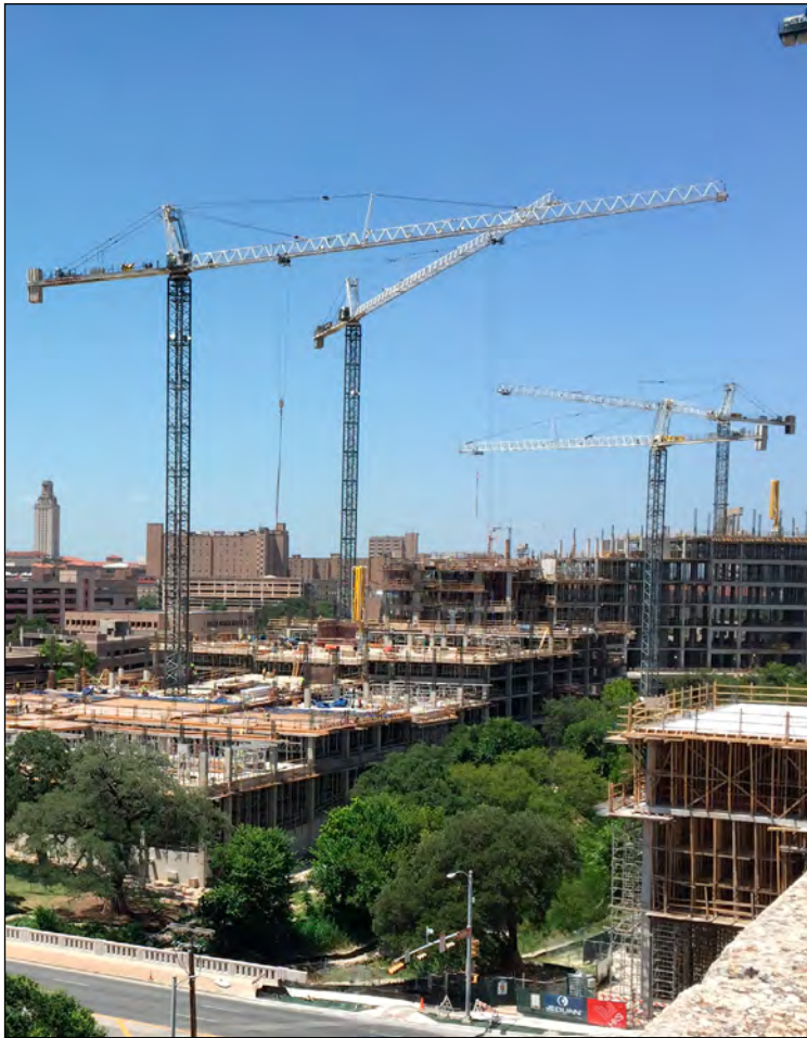
Construction of the University of Texas at Austin Dell Medical School.
