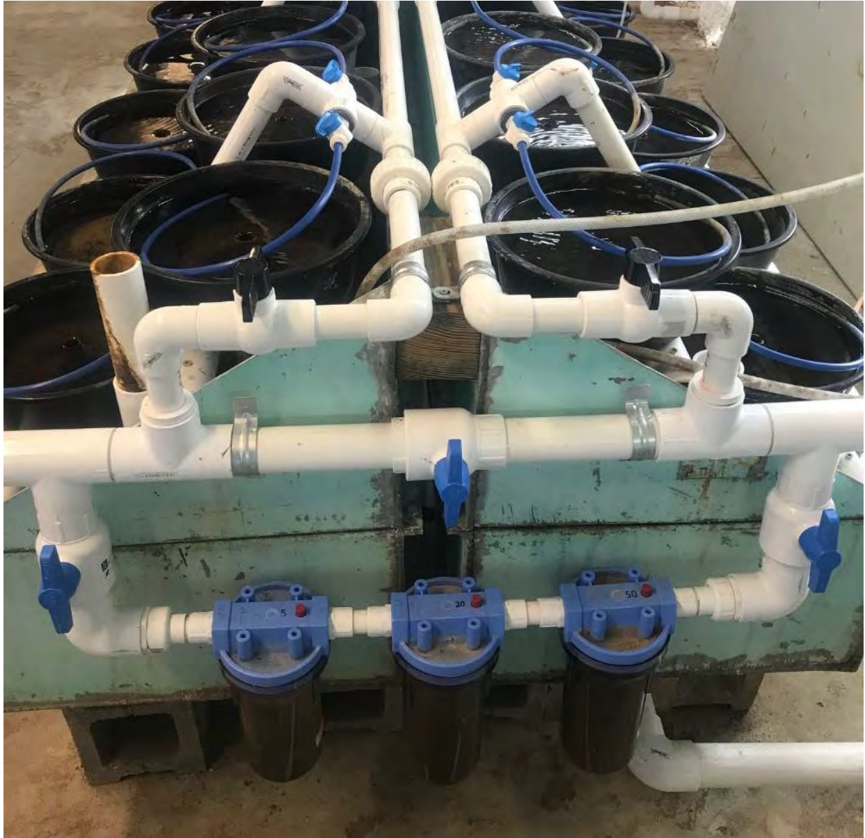
Figure 15. Paired semi-closed filtered vs. unfiltered pan systems. Photo Credit: USFWS
