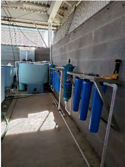
Figure 4. Recirculating (AHAB) flow-through system for holding inoculated fish. Photo Credit: USFWS
