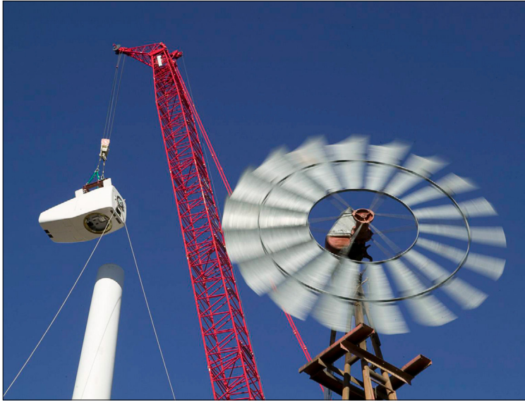
Wind Farm Construction
