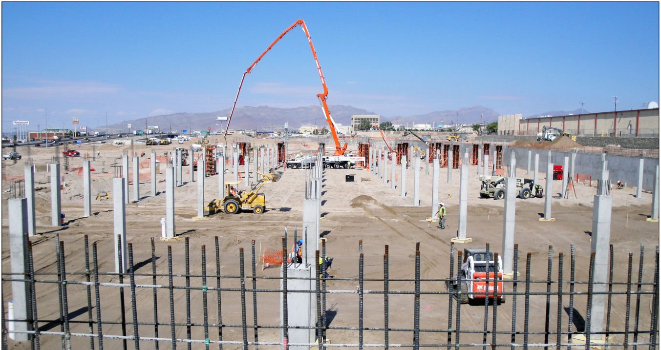
Construction of the “The Fountains at Farah” project in El Paso PHOTO: Courtesy of Centergy Retail, LLC.
