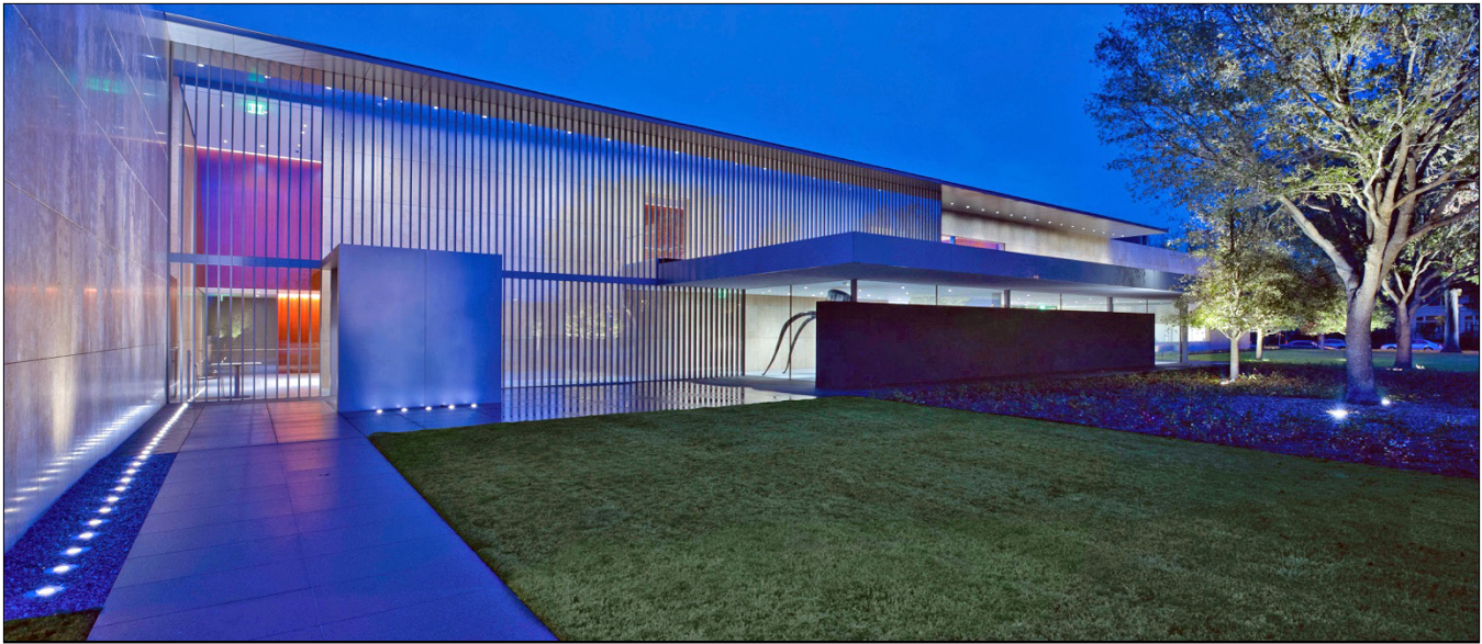
Texas Asia Society Center in Houston PHOTO: Courtesy of Greater Houston Convention and Visitors Bureau
