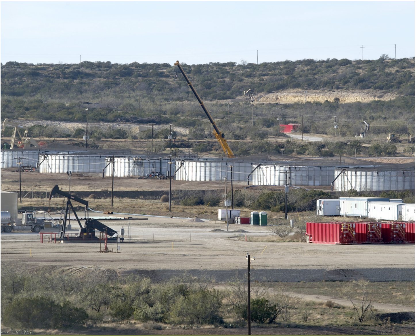
Apache stores water in converted grain bins prior to reuse.
